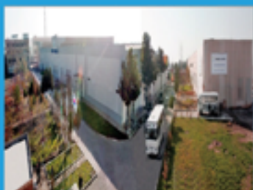
Shindong Spinning Termez LLC
